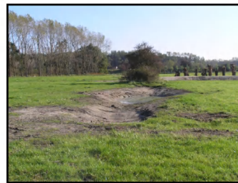
Figure 4: the jumping after the works
