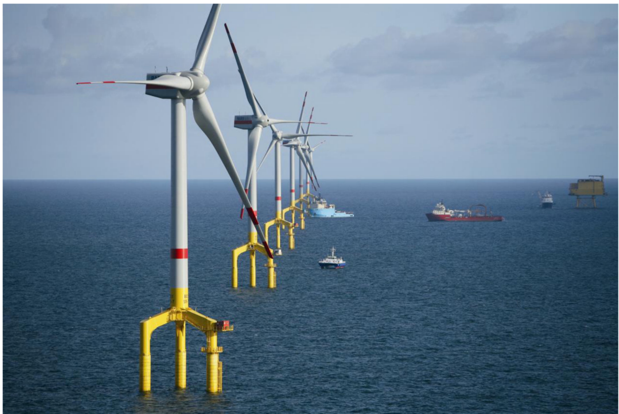
Figure 11: BARD offshore I wind park – first six turbines with tripile foundations
