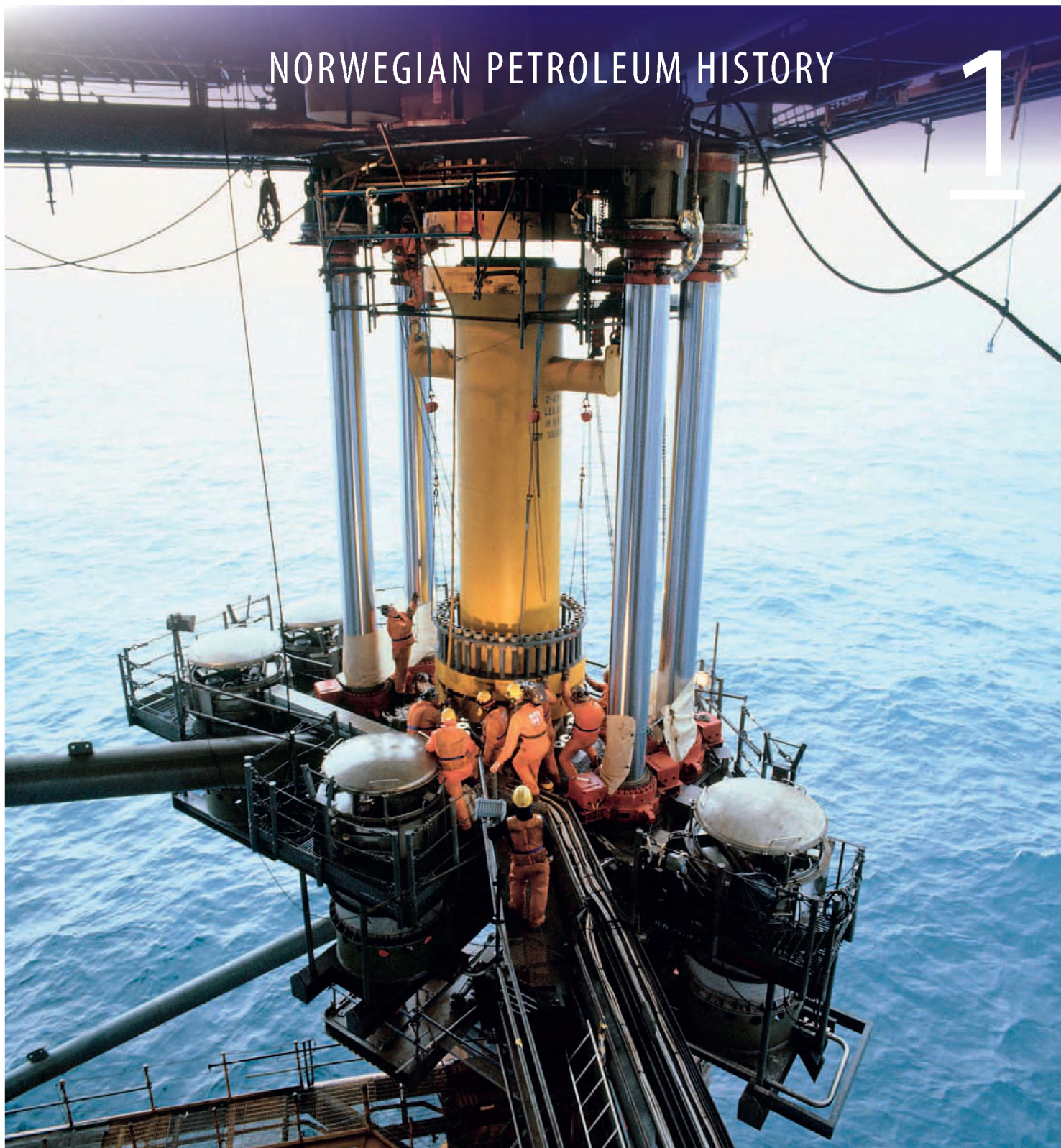
From the jacking up of the Ekofisk platforms in 1987. Here a piece is being put in place to extend one of the legs on the Ekofisk 2/4 hotel facility. (Photo: Husmo, ConocoPhillips/Norwegian Petroleum Museum)
