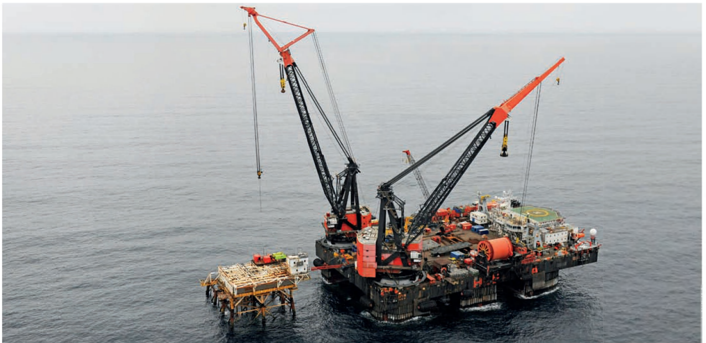
Figure 6.7 The Balder heavy lift vessel prepares removal of the Edda topside frame (Photo: Kjetil Alsvik, ConocoPhillips)
