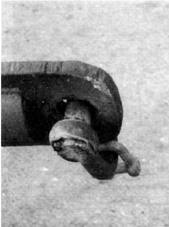
Figure 9: Padeye at lower end of spar (counterweight) showing the 25 mm shackle, with bolt welded in place
