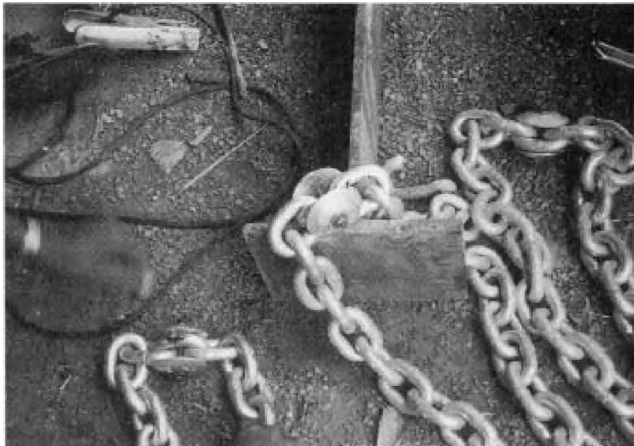
Figure 10: Tack-welding a zinc button anode to the upper chain to guard against corrosion
