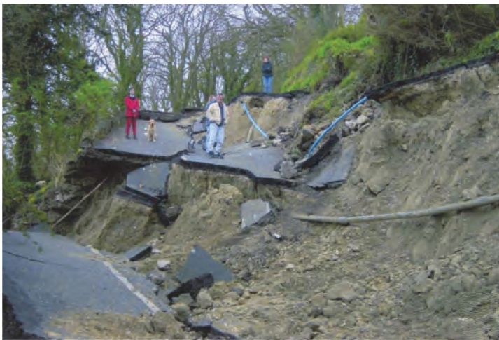
Plate 5.8: Landslide damage to A3055 coast road, Niton, Isle of Wight, UK, Spring 2001.
