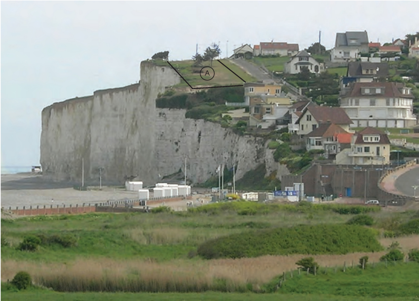
Plate 2.7: At Criel-Sur-Mer on the Channel coast of France rapid erosion of the vertical chalk cliffines has resulted in the loss of residential cliff top properties. For environmental and economic reasons coastal defence was not an option; recently a row of the most vulnerable properties (A) have been demolished under the provisions of the Barnier Law.
