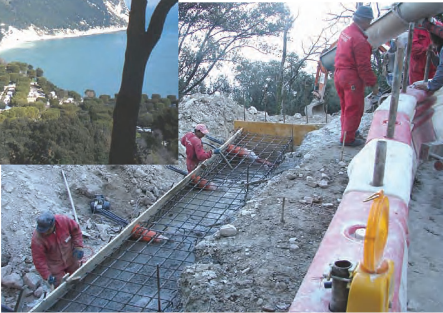
Plate 2.4: Landslide stabilisation measures including ground anchors assist in reducing risks on the seaward slopes below the historic town of Sirolo, Marche Region, Italy.
