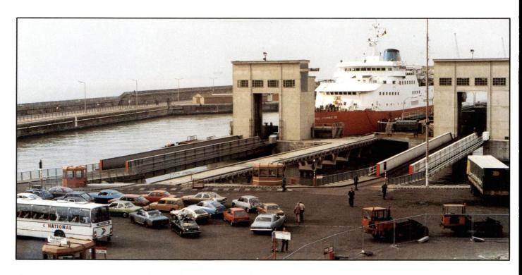
Both main bridges rest on sliding hinges on the land side. They are slug in cables with counterweights and can always be lifted immediatly, even during power cuts. The lifting speed is 0.20 m/sec.
