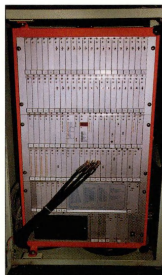
Central computer for monitoring the incinerator system and registering the parameters
