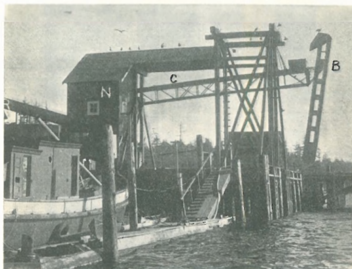
Fig. 3. The unloading machinery and control-room at Ucluelet. (B) Marine leg; (C) pivoted conveyer; (R) fixed conveyer; (N) control-room for tag recovery equipment.
