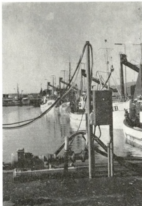
Fig. 5. Pump for bilge water.
