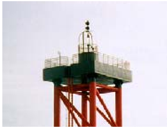
Fig.3 Chuluncho light beacon station
