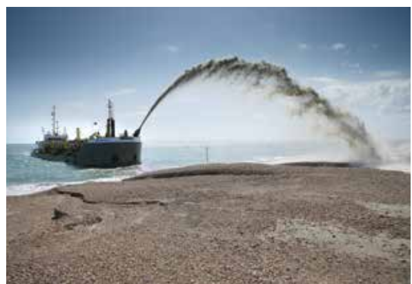
Fig 1.2 Pumping material onshore, © Westminster Dredging Company Limited.
