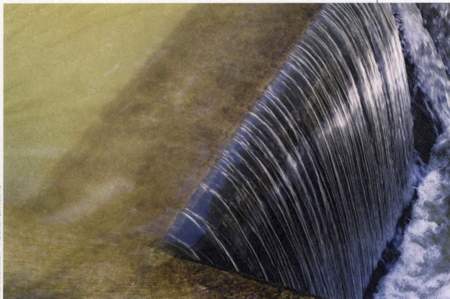
RWZI DIKSMUIDE – WOLMEN (EFFLUENT)
