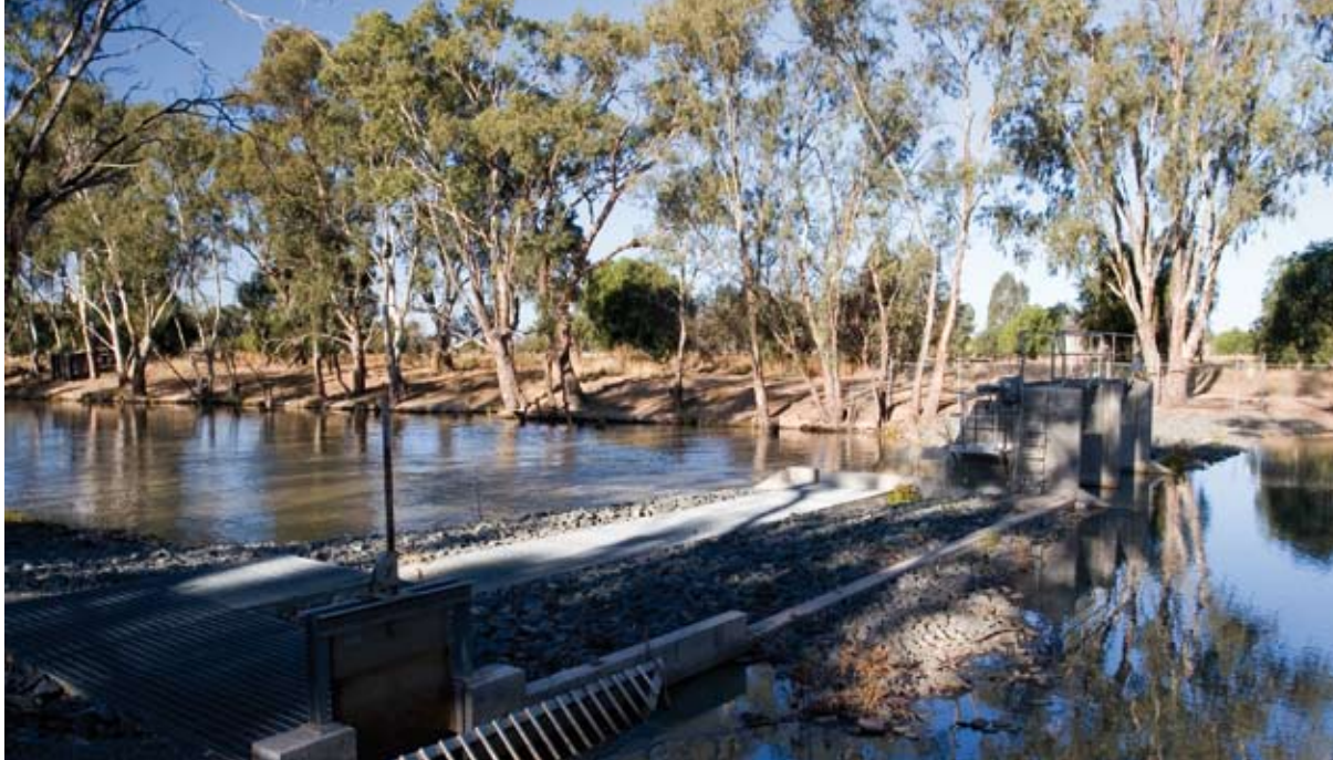
Fish ladder on Broken River weir, Nathalia, Victoria. In some river systems fish ladders can overcome a range of problems. However other issues such as river flow and temperature profile remain problems. Photo: J Baker, DEH.
