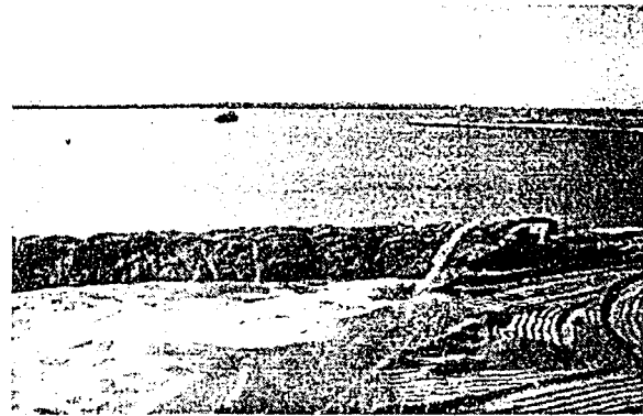
Fig. 3. Nourishment works on Aculadero beach, with the pipeline pumping sediment on to the beach. Note the dredging boat in the background.
