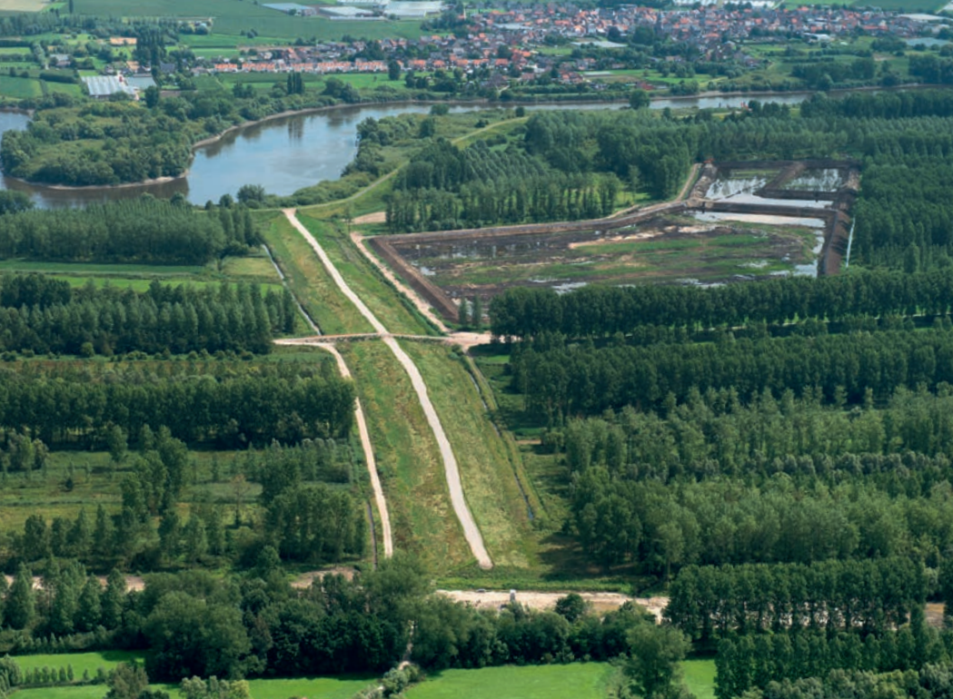
Figure 23. The completed overflow dyke in autumn 2013, covered with vegetation for protection against erosion.
