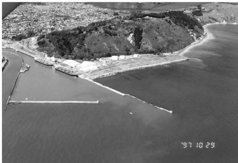
Fig. 3. Port outlay and present area of log storage. For redesign the reclamation is planned to extend along the shore platform, and the right breakwater will need to be removed.
