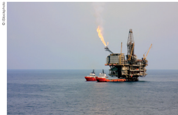
Figure 6.3. Offshore oil platform with support ships
