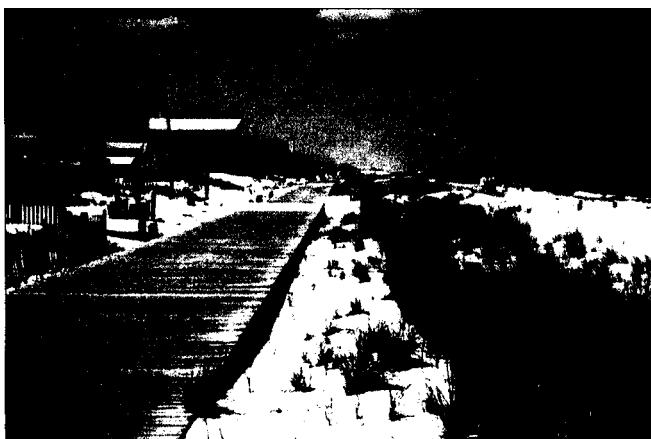
Figure 2. Dune at Lavallette, New Jersey, showing a dune built as a sand dike primarily for protection on a shore where beach space prevent restoration of a large fully-functioning dune.
