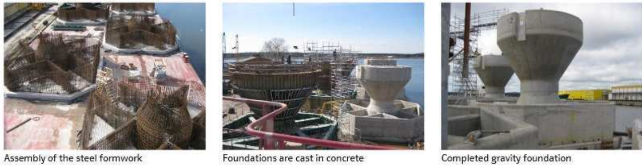
Figure 25. Manufacture and delivery of Gravity base foundation (EON, 2012)
