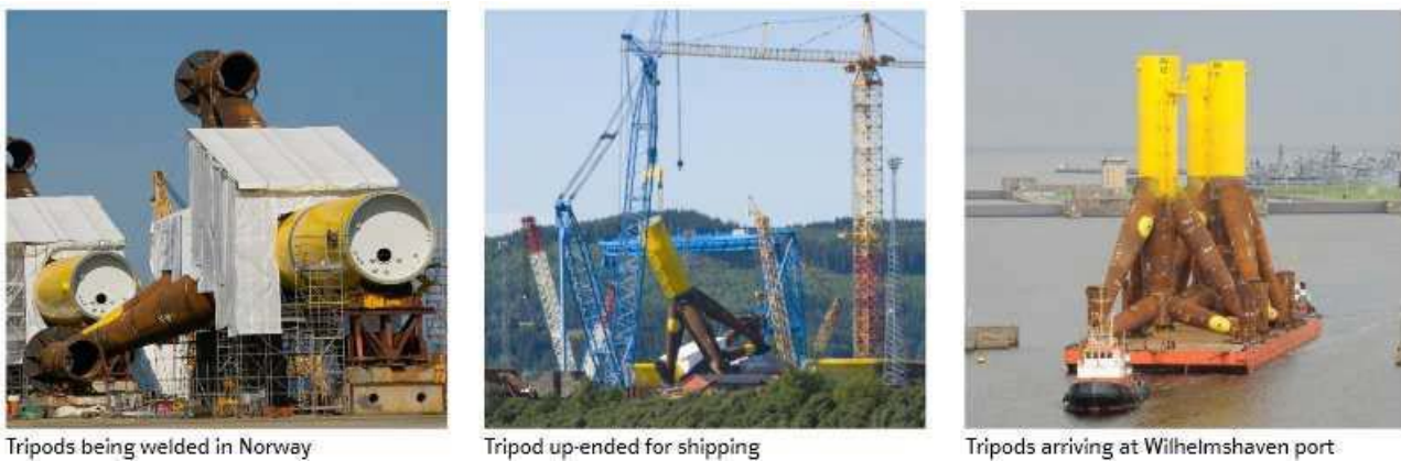
Figure 29. Manufacturing and delivery of tripod foundations (EON, 2012)
