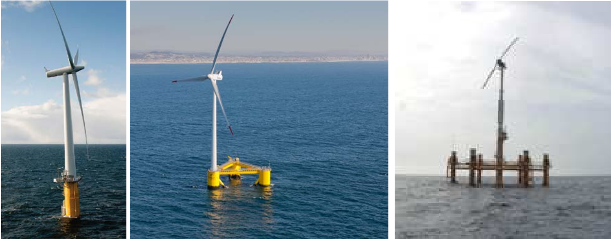
Figure 78. Prototypes developed in wind energy sector: (a) Hywind (Statoil). (b) Windfloat (Principle Power). (c) BlueH TLP (BlueH)
