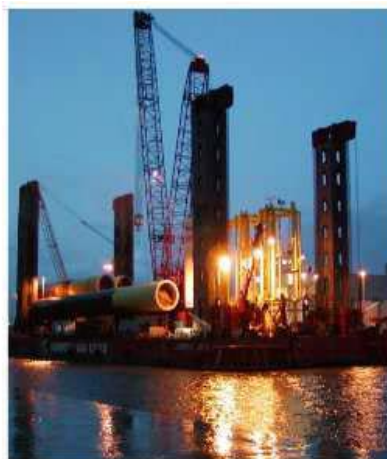
Monopiles loaded out on jack-up barge
