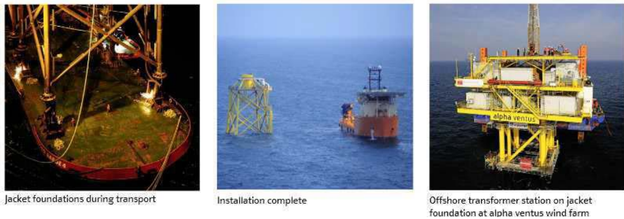
Figure 28. Installation of jacket foundation (EON, 2012)
