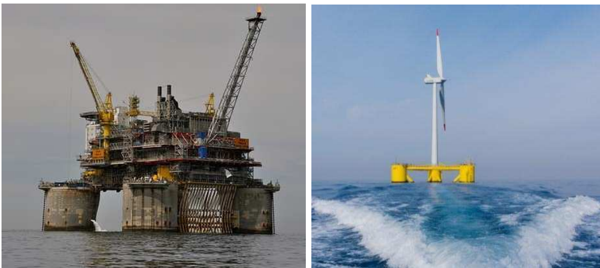
Figure 13. Semi-submersible structures: (a) TROLL B (North Sea, 1995); (b) WINDFLOAT 2MW Phase I, Installed 2011
