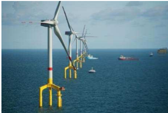
Figure 31. The Bard 5.0 MW turbines, supported by tripile structures at 40 m water depth at the offshore plant 'Bard Offshore 1'. Photo: Bard Offshore
