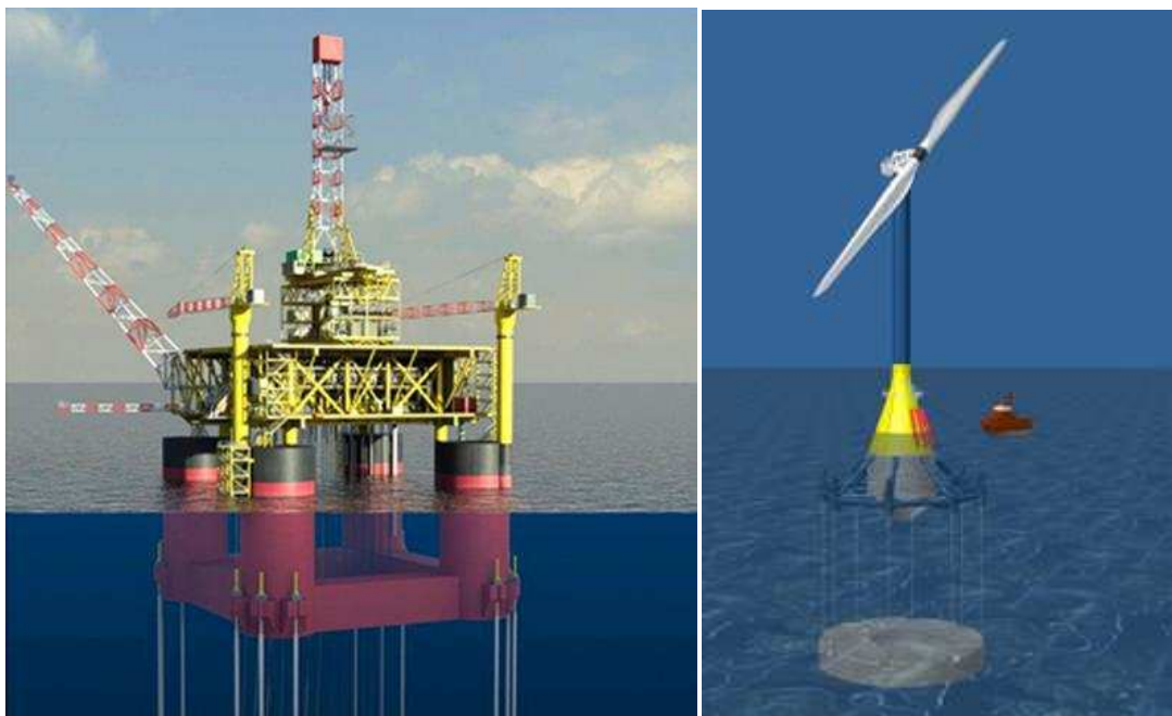
Figure 18. TLP concept. (a) HYUNDAI TLP structure for Oil&Gas. (b) Blue H TLP concept for wind energy
