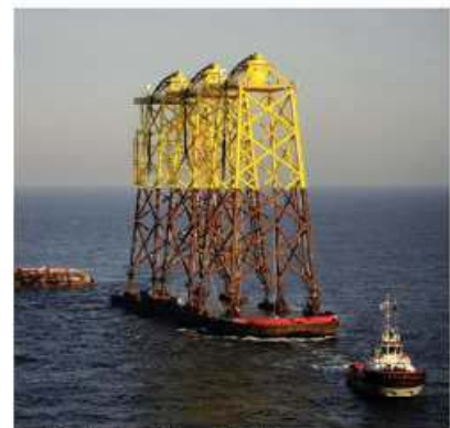
Jackets being shipped to site
