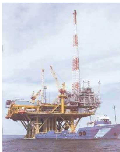
Figure 4. COGNAC Platform installed in deepwater Gulf of Mexico (Source: Offshore Magazine)
