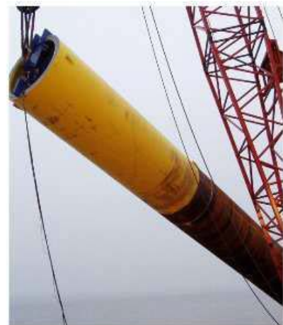
Monopile being up-ended for installation
