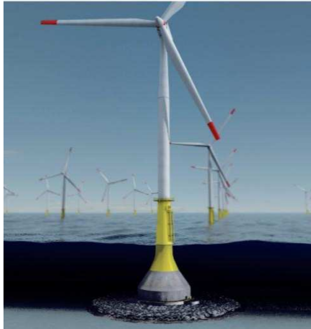
Figure 55. Cranefree Gravity (CFG) foundation
