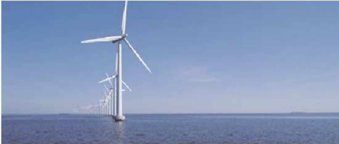
Figure 53. Middelgrunden offshore wind farm Denmark
