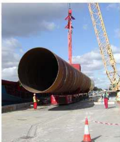
Monopile delivered to harbor
