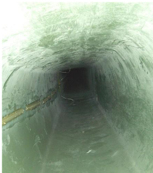
FIGURE 3.3 The middle (of the three) compartments inside a turbine blade. Source: [15]
