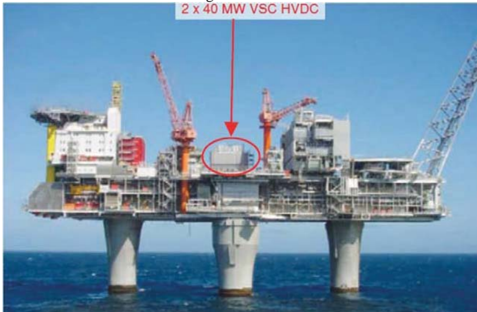
Figura 79 - VSC power supply to Troll A production platform [source: ABB].
