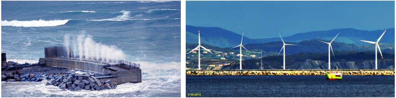
Figure 22. Different combined uses: Break water + OWC or Wind Turbines: [20].
