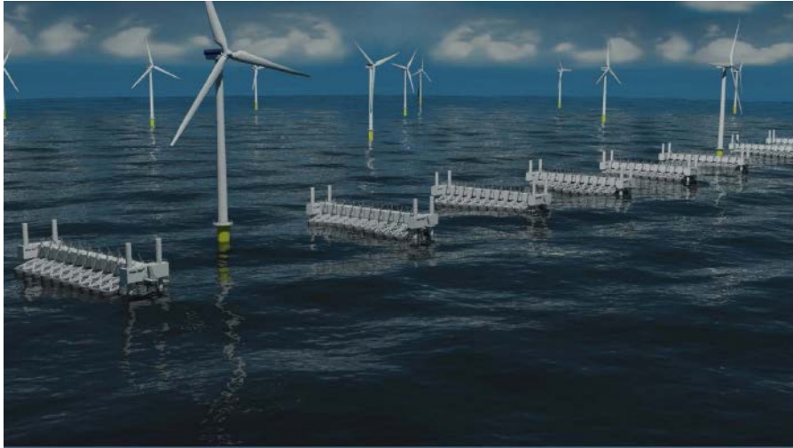
Figure 20. Multi-purpose offshore farm: Sharing space concept: Wind Turbines + Wave Star [19].
