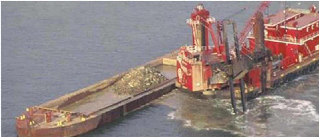
Figure 2.2 Offshore dredging works
