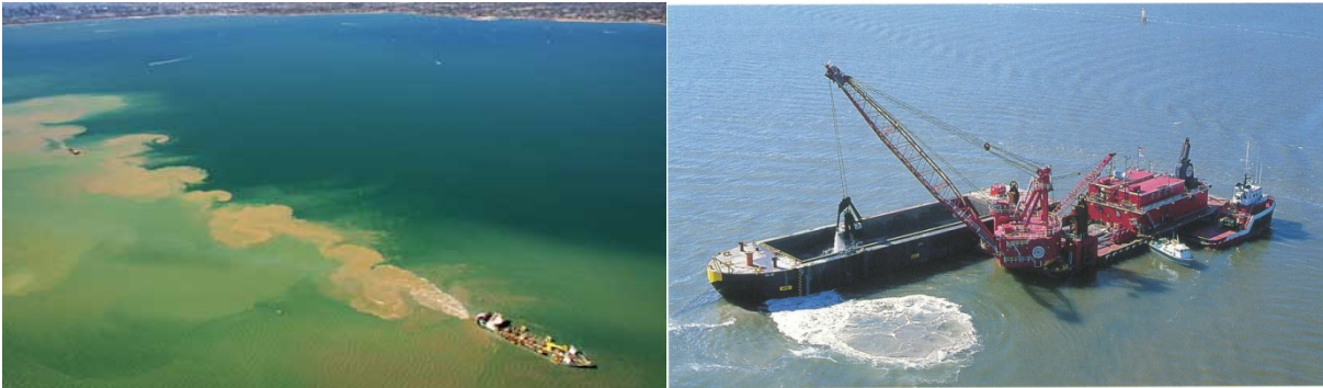
Figure 2.6 Left: Overflow plume, Right: Spill from the grab
