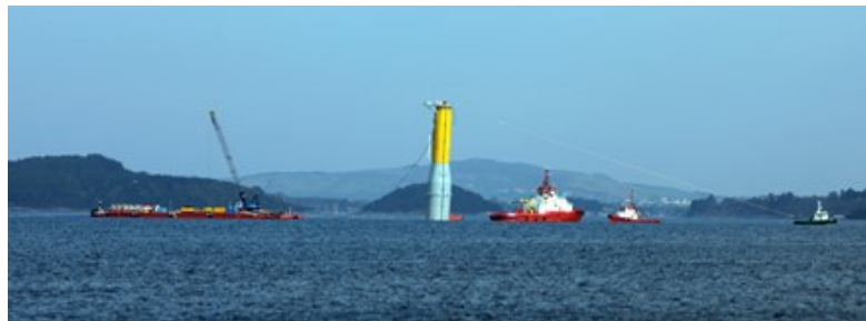
Figure E.5 Hywind Demo up-ending of the sub-structure in Åmøyfjorden
