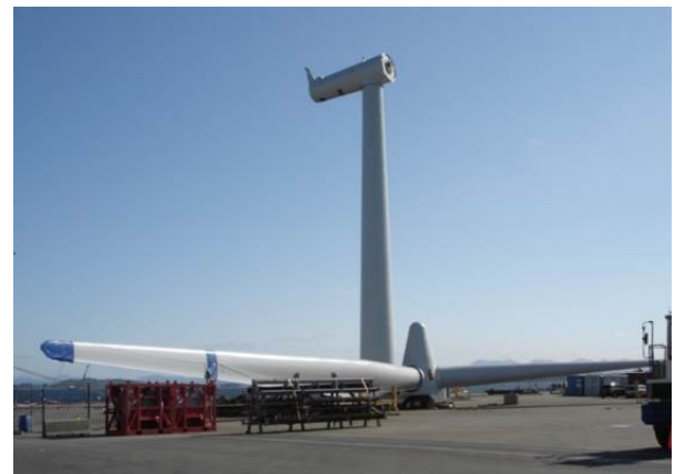
Figure E.6 Rotor with hub, upper tower segment and nacelle on the quay at Dusavika
