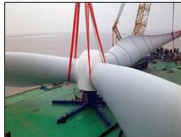
Assemble rotor on the vessel
