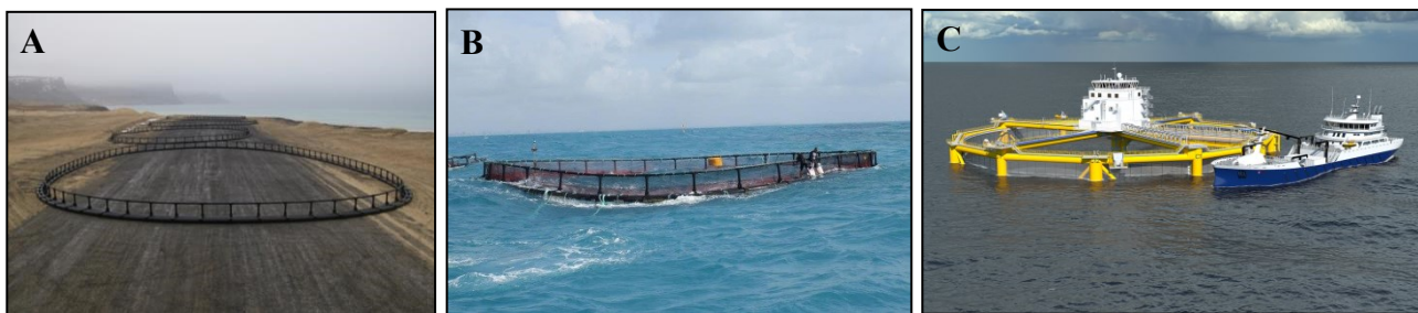
Figure 2.17 Fish cage assemble onshore (A); Fish cage operation offshore (B); and next generation strong fish cage (C)
