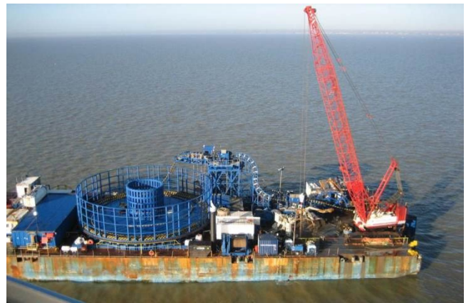
Figure 2.14 Cable installation barge with turntable.
