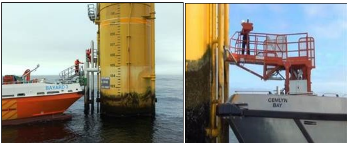
Figure 2.21 Current push-vessel-against-foundation method for assessing WTGs
