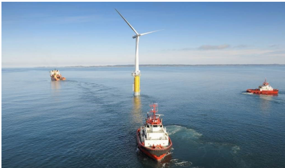
Figure E.10 Vessels used in the tow-out from the inshore assembly site.
