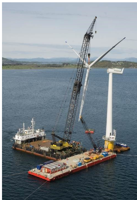
Figure E.9 Rotor lifted onto the nacelle using Conlift
