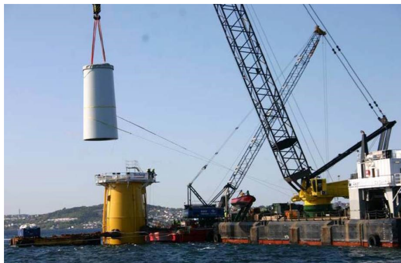
Figure E.7 Assembly of lower tower section
