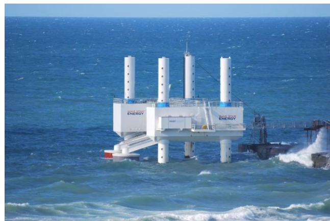
Figure 3.5.6 – To the left, the principle of operation of the Wave Star. To the right, a Wave Star prototype (with only two floaters) installed at Hanstholm (DK).
