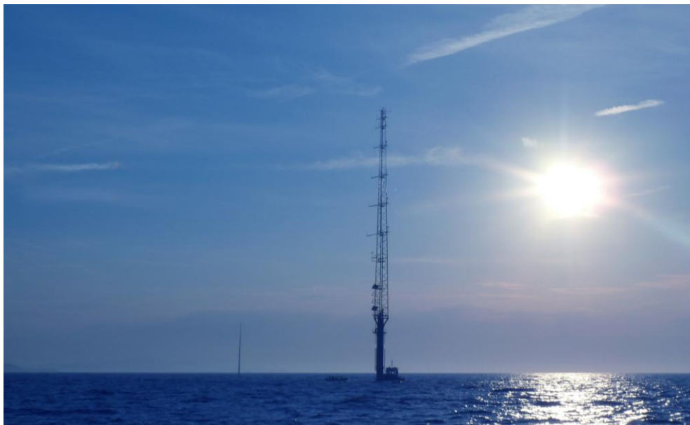
Figure 2.3.6. Idermar floating met mast at Cantabrian Offshore Site
