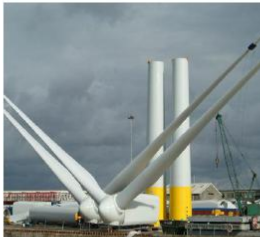
Figure 3.2.7 - Pre-assembled turbine parts in the harbor.
