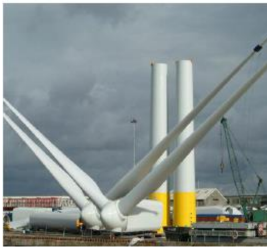
Figure 5-9 Pre-assembled turbine parts in the harbour.
