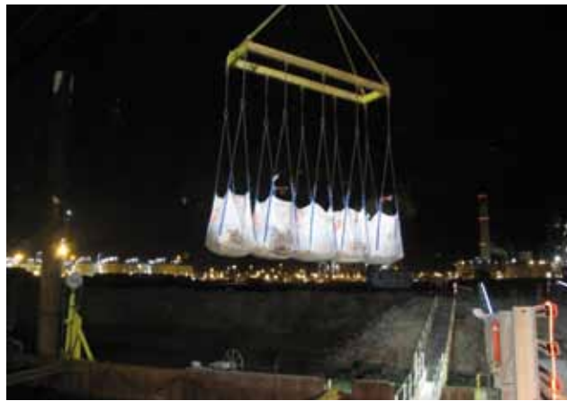
Fig. 2.23. At the end of each working day the dredger Triton unloaded the bulk bags onto the quay.
