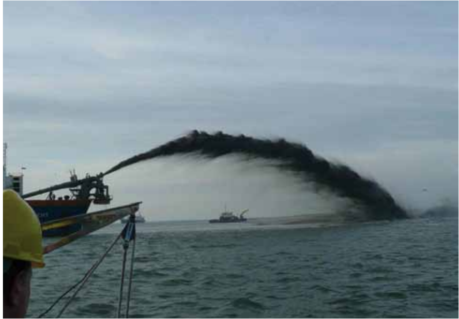
Figure 2. Rainbowing of the extracted sediment to create new land. Photo: Th. van Kolschoten.
