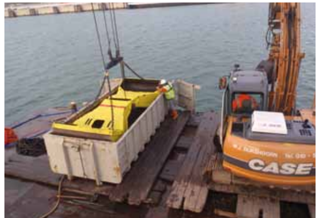
Fig. 2.18 If river-dune deposits were encountered in a soil sample, it was dumped into a container on board the pontoon.
