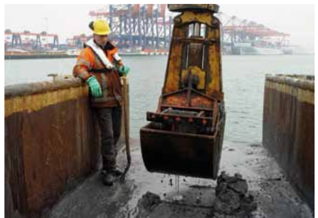
Fig. 2.20. A backhoe with a small hydraulic grab scooped the soil sample out of the container.
