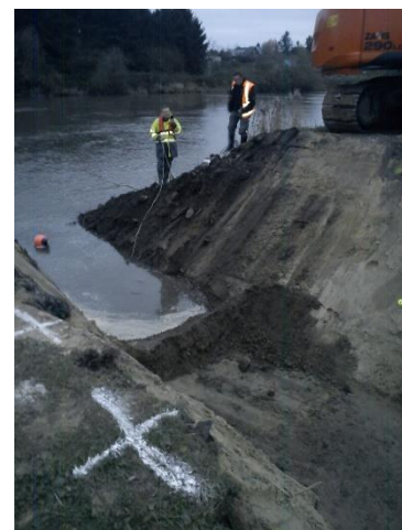
Figure 4-4 Pilot channel before test
