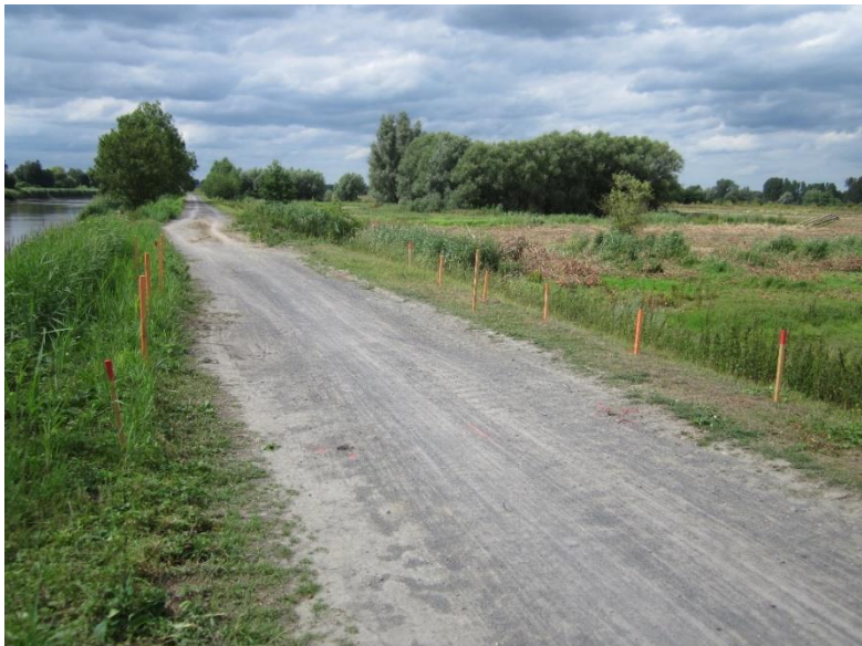
Figure 1-5 Dike at location breach experiment
