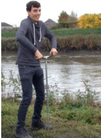
Figure 4-2 Installation of sensors using an auger
