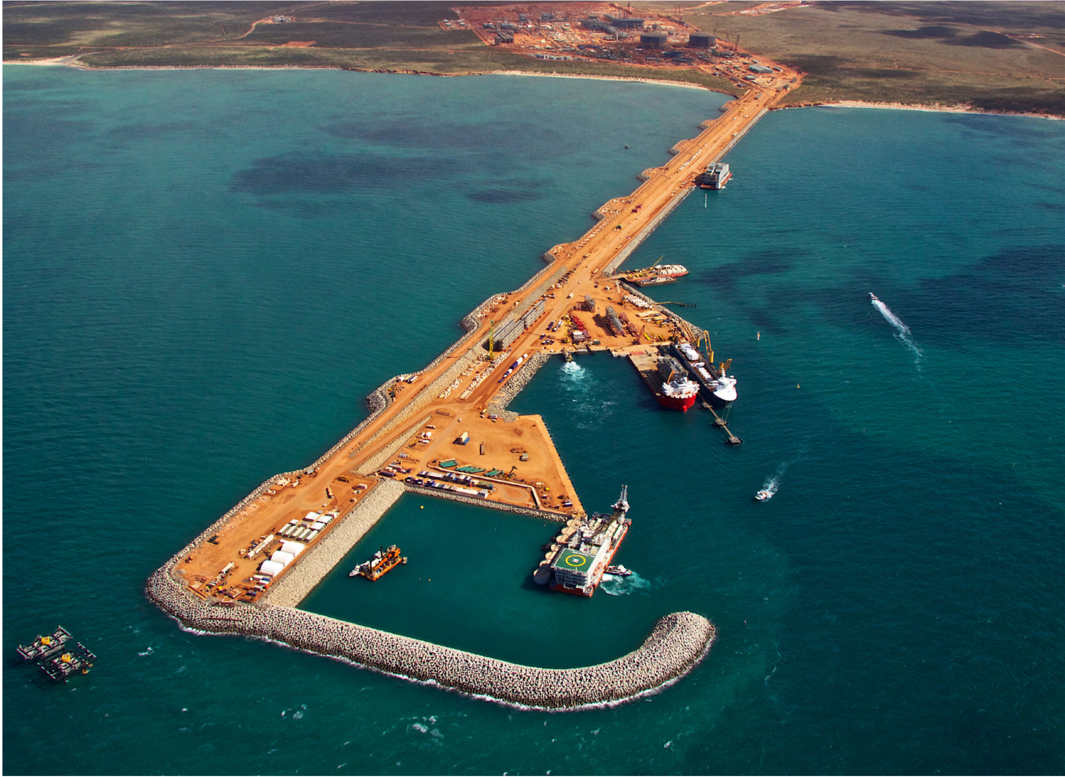
→ The remote location and the limited accommodation on Barrow Island during the work resulted in chartering a Marine Construction Support Vessel to accommodate up to 400 staff and workers. ← Aerial view of the jetty at Barrow Island near the Gorgon LNG fields comprising a material offloading facility, quay walls, mooring dolphins and a roll-on/roll-off facility.
