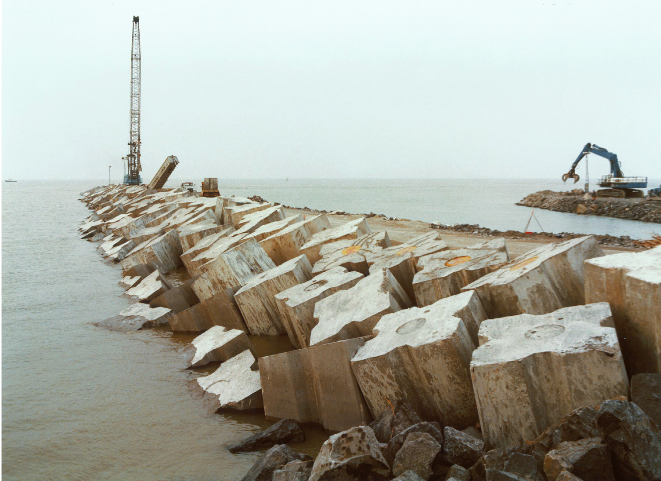
↑ Aerial view of the breakwater and reclamation works. ← 11 million tonnes of quarried rocks and 60,000 concrete armour units were installed for the rock revetments and breakwaters at Zeebrugge.
