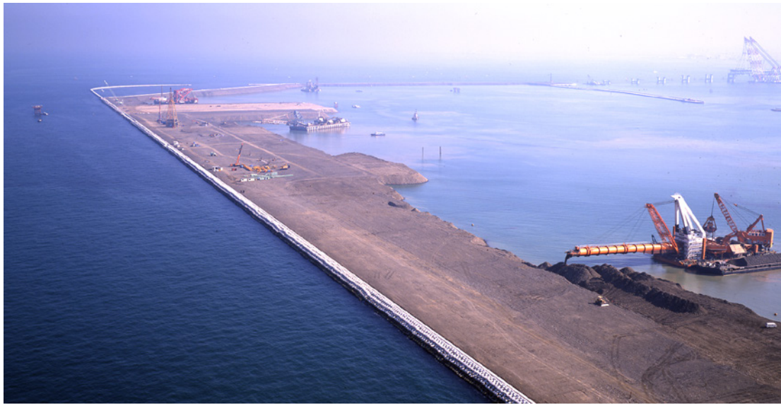
Early stages of the land reclamation for Kansai airport in Osaka Bay.
