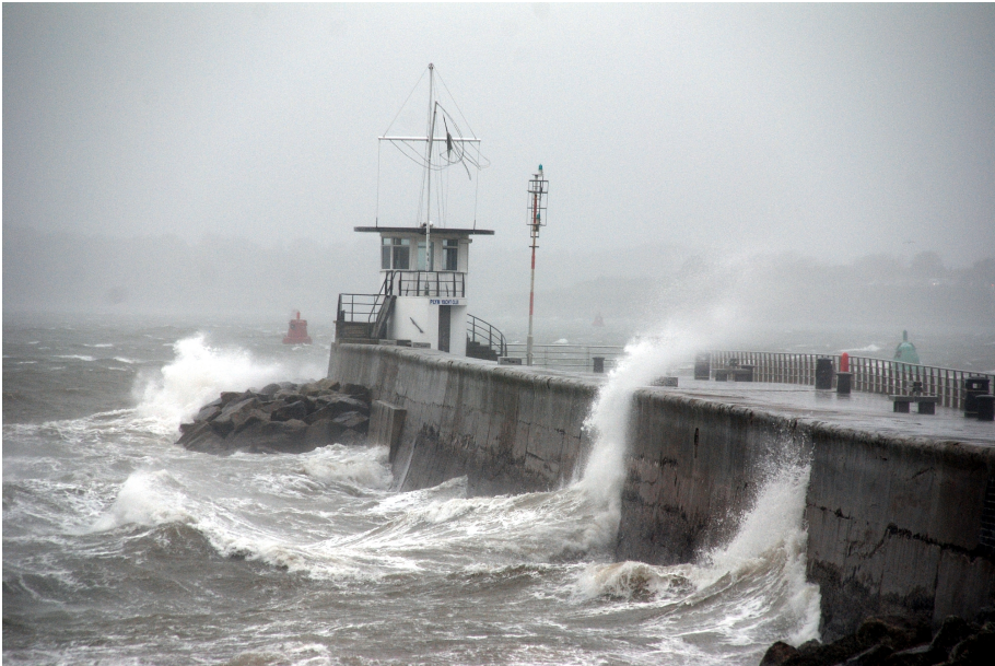
Figure 1.3: Vertical breakwater during a storm event in 2012 (Mount Batten, UK). Photo: Declutter
