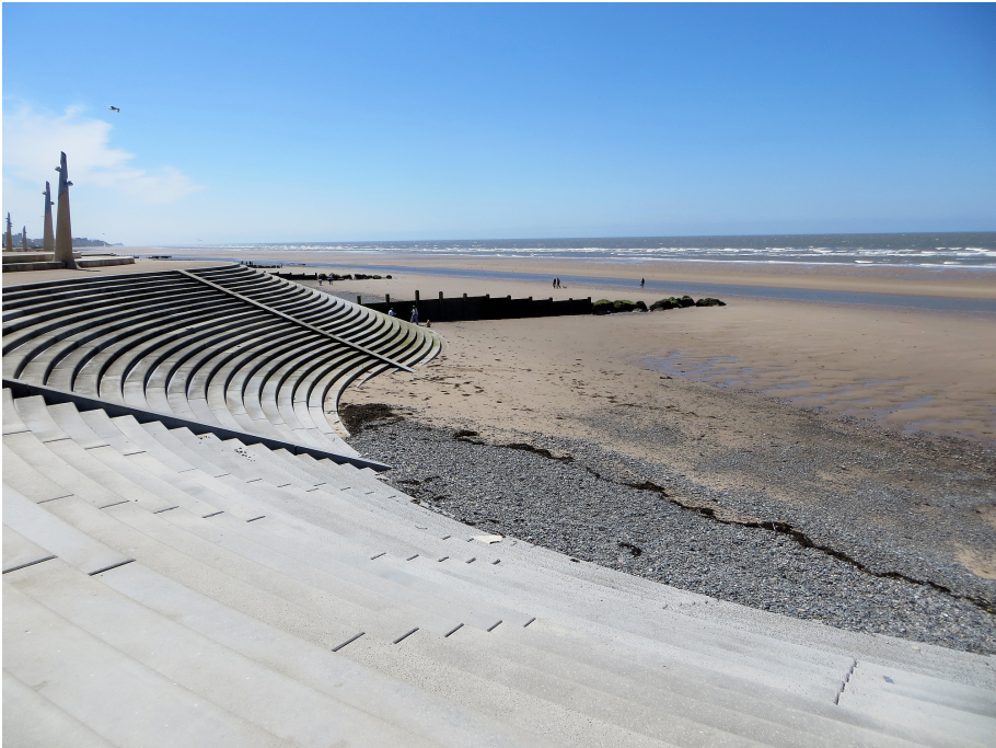
Figure 1.4: Stepped revetment as coastal protection in Cleveleys (UK). Photo: Philip Platt.
