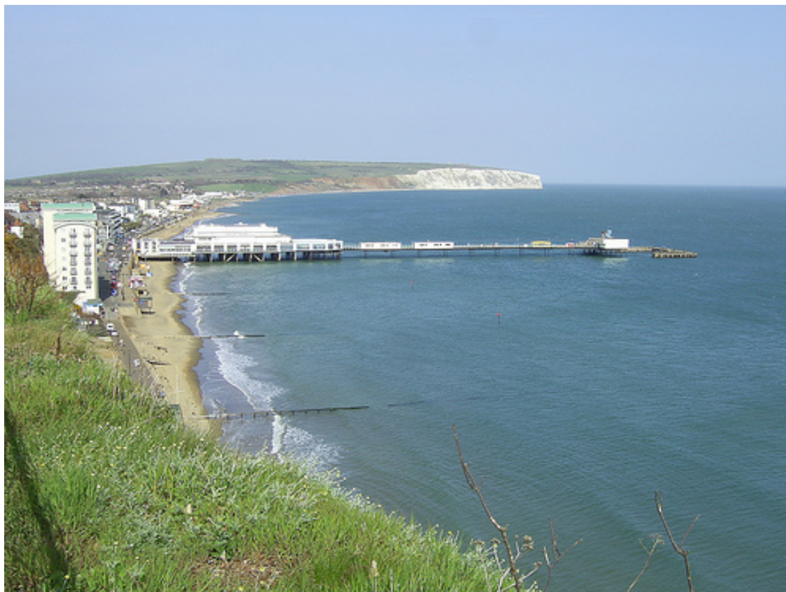
Figure 8.25 The vista across Sandown Bay as viewed from the south demonstrates the vulnerability of the low lying urban development to changes in the land-sea relationship. Coastal instability is not uncommon around the bay. The cliff from which this image was taken is under constant attack from the sea and has been subject to landfalls (R & G Long)
