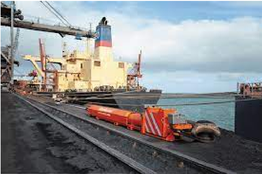
Figure 2.22: Application of ShoreTension at a berth, from ShoreTension website.
