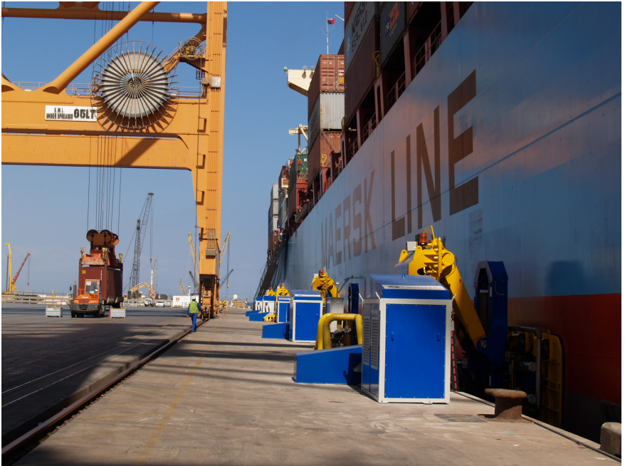
Figure 2.23: Application of Cavotec MoorMaster at a berth, from Cavotec website.
