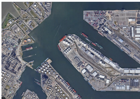
(c) Sheltered Terminal, Google Earth.
