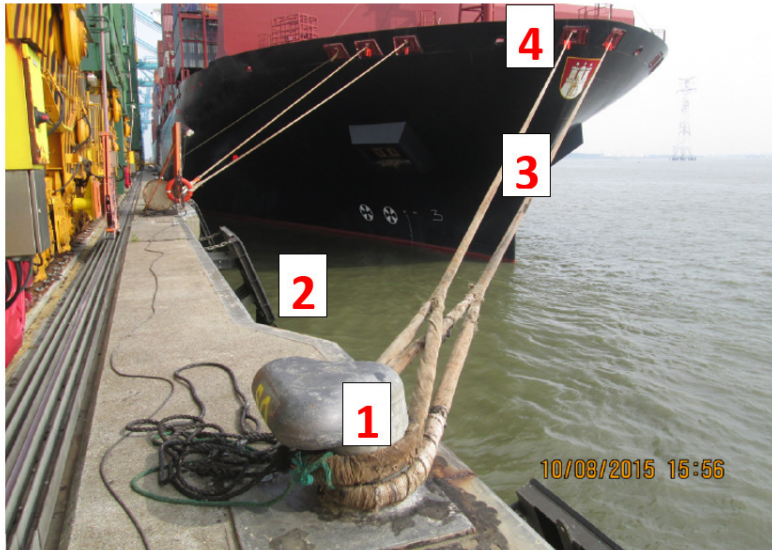
Figure 2.11: Overview mooring equipment (I), (1) bollard, (2) fender, (3) mooring line, (4) (roller)fairlead; image courtesy of Antwerp Port Authority
