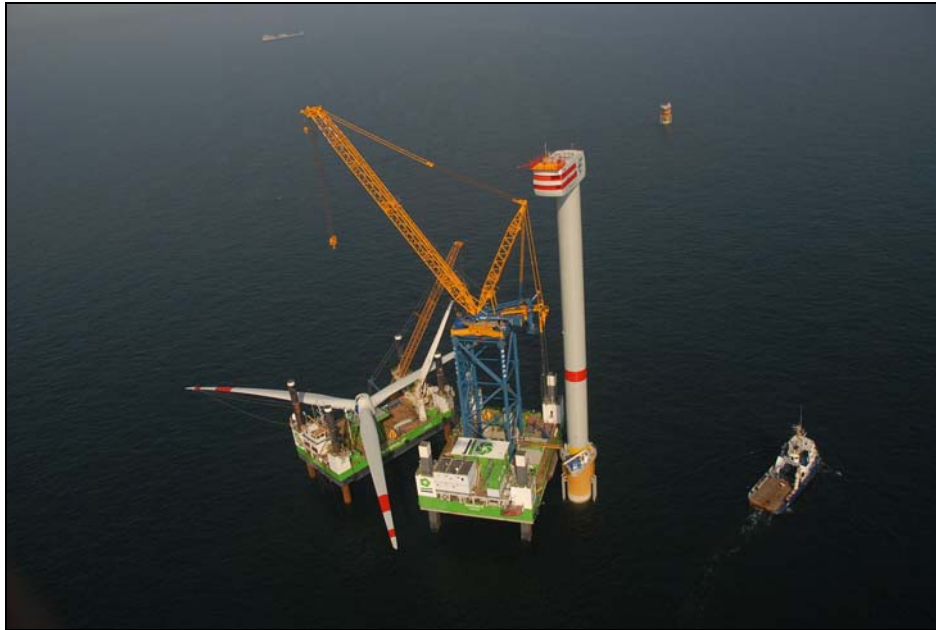
Figure 5. Installation of a turbine on the Thorntonbank (Photo RBINS).
