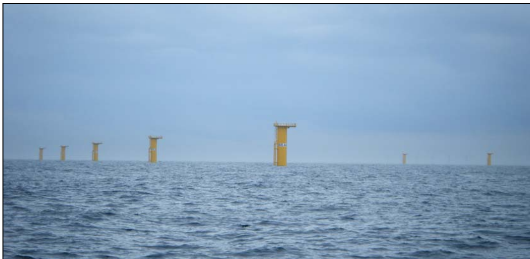
Figure 11. Installed MPs with transition pieces (yellow) on the Bligh Bank (Photo RBINS).
