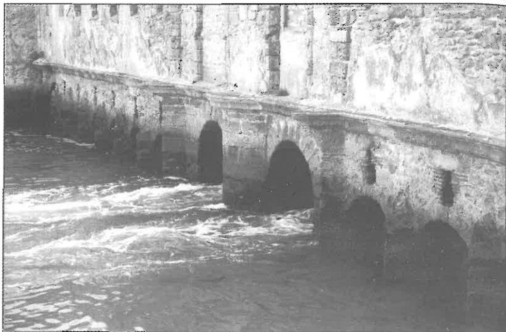
Fig. 11. The main façade of the Arillo Mill (Cadiz, Spain). Water flowed into the pond through eight entrance sluices: four on main façade and four others perpendicular to the mill (not seen here); the most important are behind the two larger central arches. All the exit sluices are on this main façade. (Photo Loïc Ménanteau, November 1991).
