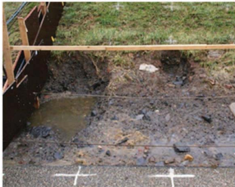
Figure 39: Damage after 5 tests with various Ru_{2\%} -levels
