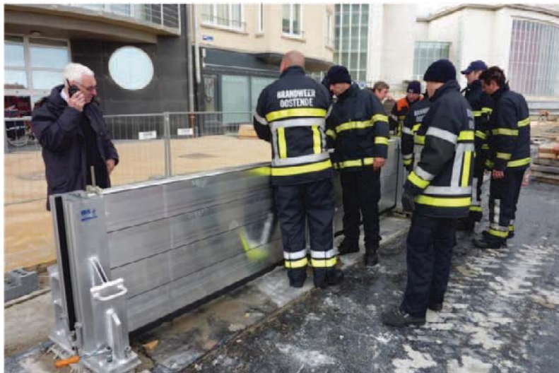
Figure 4: Firemen setting up the mobile storm wall.
