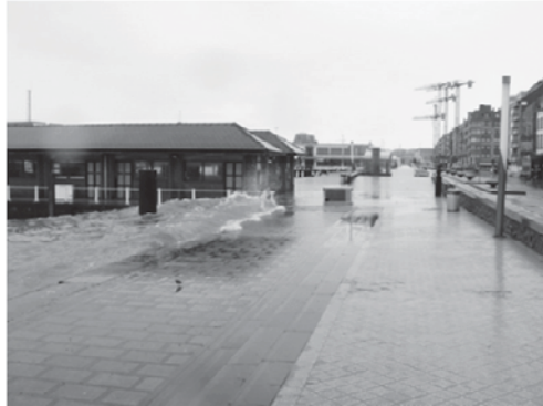
Figure 1: Water reaches quay crest level during a 5-year storm in the harbour of Oostende.
