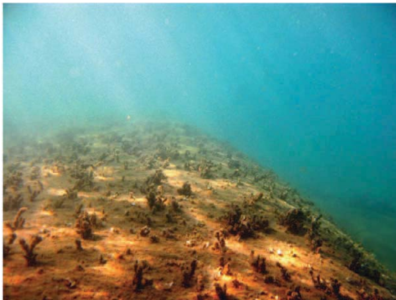
Figure 6: Geotextile tube surface 13 months after installation [Mori]
