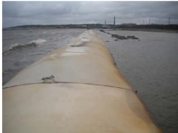
Figure 1: Geosynthetic tubes as containment bund for land reclamation
