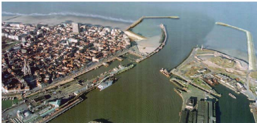
Figure 1: Artist impression of the new harbour entrance in Oostende, Belgium (works in progress).
