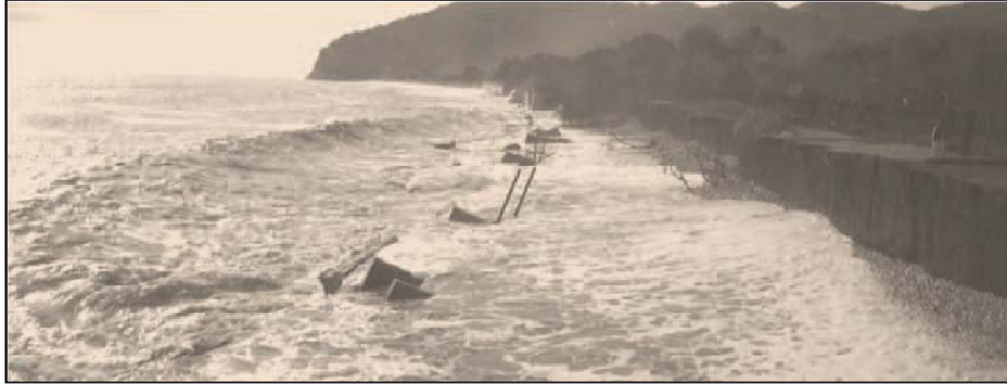
Figure 4: The waves of the storm of 28 th and 29 th of December 2002 completely eroded the beach and over the walls that border private property.
