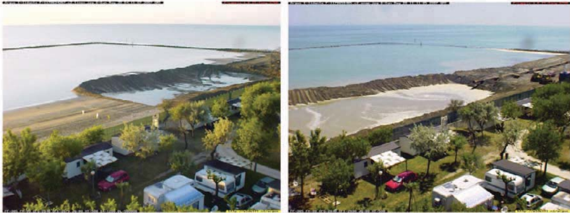
Figure 1: Snapshot images of the 2007 nourishment intervention at Lido di Dante taken from the ARGUS video station.
