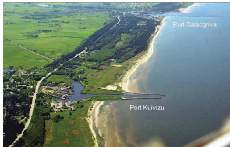
Figure 3: Aerial photography of the project sites
