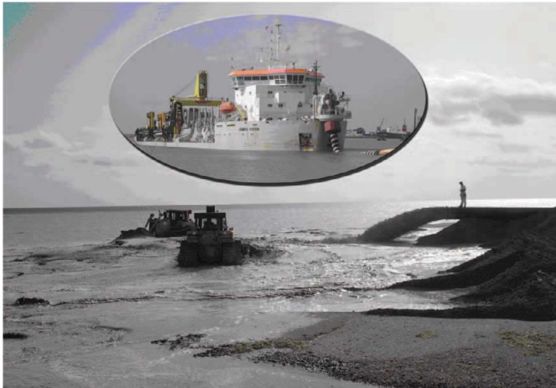
Figure 7: Photos of the dredger and the ongoing hydraulic fill
