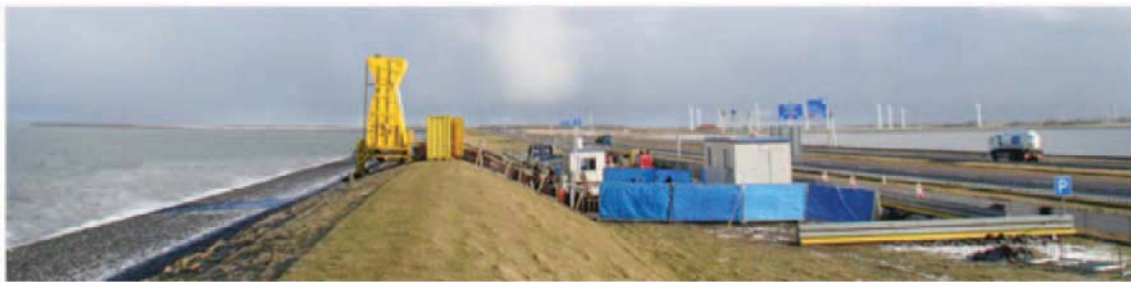
Figure 18: Set-up of Wave Overtopping Simulator close to a highway (February 2009).
