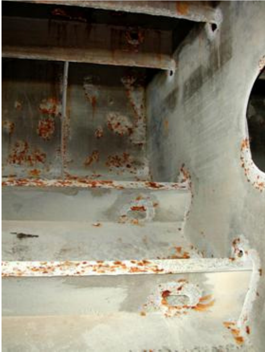
Figure 111: Effective anodes (Amtec, 2008)
