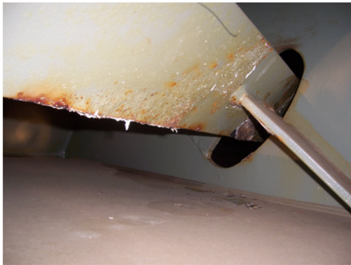
Figure 91: Effect of the presence of sacrificial anodes on the condition of the coating. Photos courtesy of Hempel.
