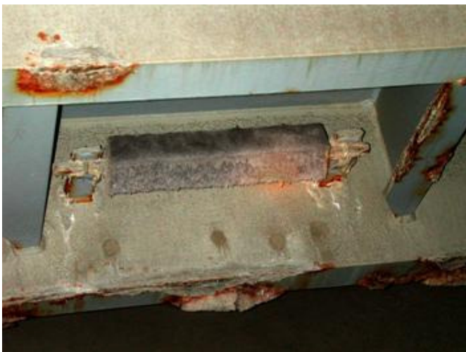
Figure 110: A poorly sited anode (Amtec, 2008)
