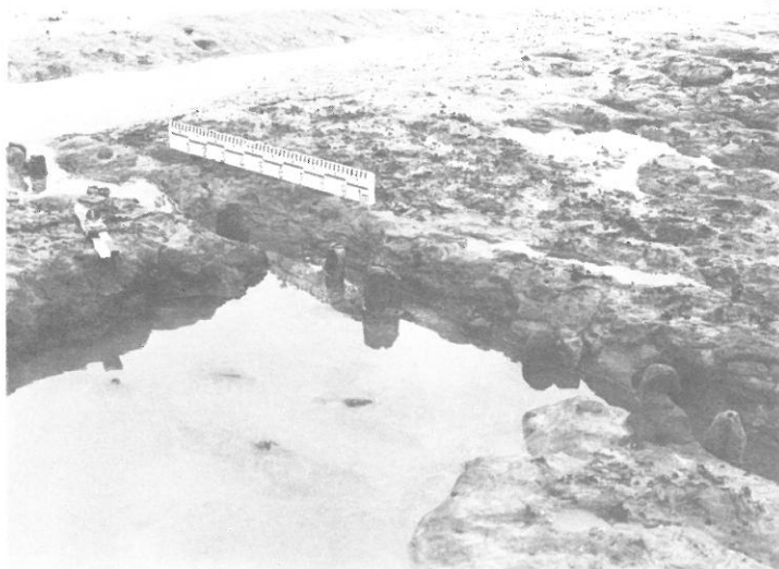
Fig. 35a. Vertically driven-in piles of a wooden saltern construction on the beach.
