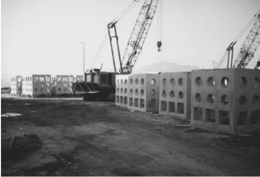
Fig. 2. Representative of efforts to incorporate biological design criteria into the physical structure of artificial reefs is the Box Reef, with open space in its upper level and confined space below (photograph courtesy of C. Kim).
