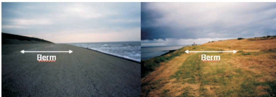
Fig. 5.28: Typical berms (photo: SCHÜTTRUMPF)
