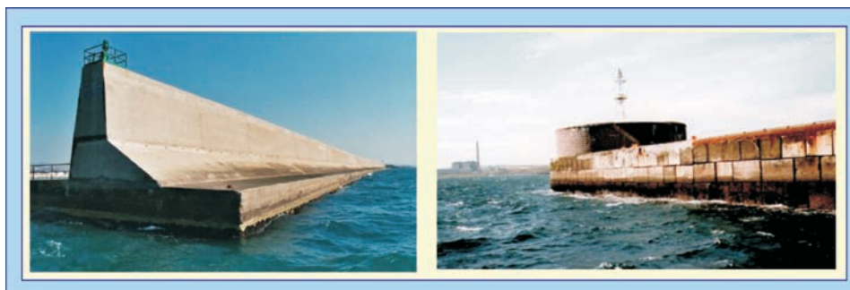
Fig. 7.1: Examples of vertical breakwaters: (left) modern concrete caisson and (right) older structure constructed from concrete blocks
