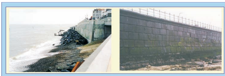
Fig. 7.2: Examples of vertical seawalls: (left) modern concrete wall and (right) older stone blockwork wall
