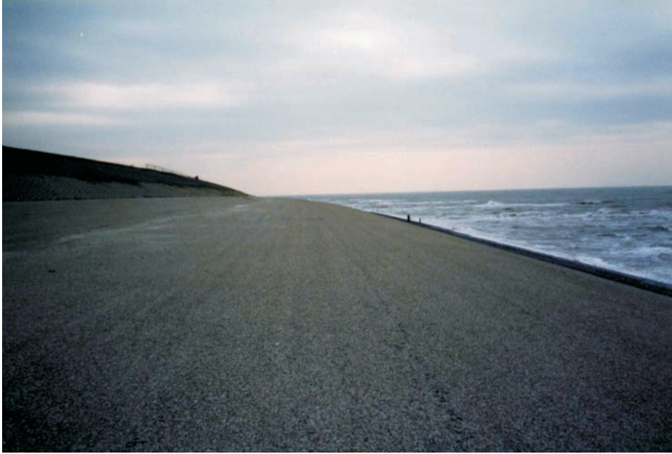
Fig. 5.16: Dike covered by asphalt (photo: SCHÜTTRUMPF)
