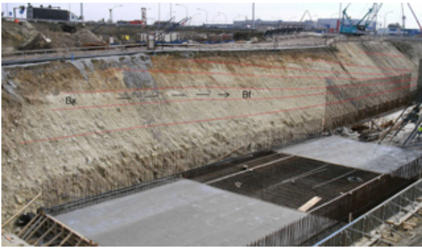
Figure 8. ESE-ward dipping bedding planes exposed in a construction pit in Machelen near Zaventem airport. Some bedding planes are highlighted in red. Here, facies Bx grades laterally into Bf. The bedding plane slope decreases in a downdip direction. Construction works of the Diabolo high-speed railway link to the airport, near Machelen exit on the E19, exposed in March 2009.
