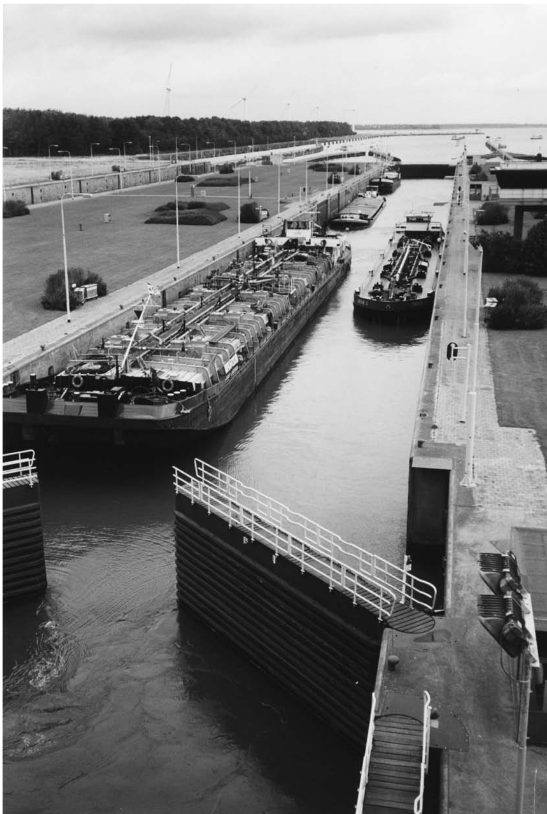
Photo 1.1 Pushtow navigation locks in Volkerak (October 1999)
