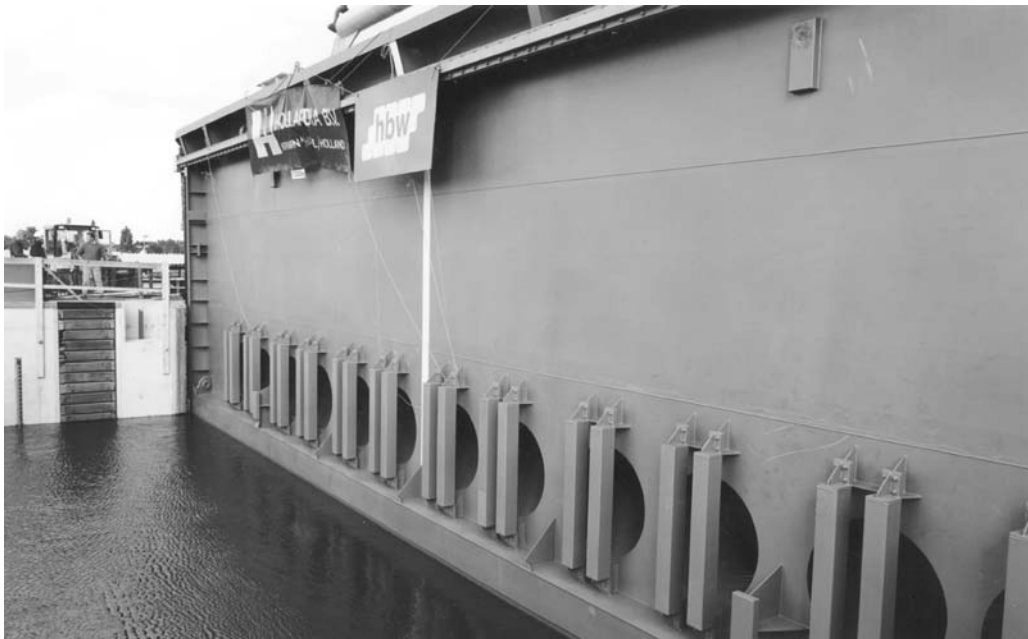
Photo 6.13 Energy dissipating bars behind the round openings of the sliding gate of Nieuwe Oranje lock in Amsterdam
