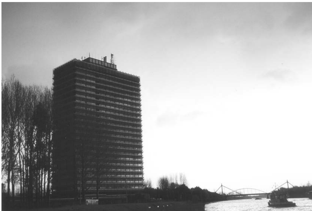
Photo 3.1 Civil Engineering Division, Utrecht branch
