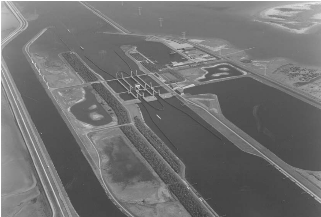
Photo 5.3 Lay out of Kreekraksluizen in the Schelde-Rijnverbinding
