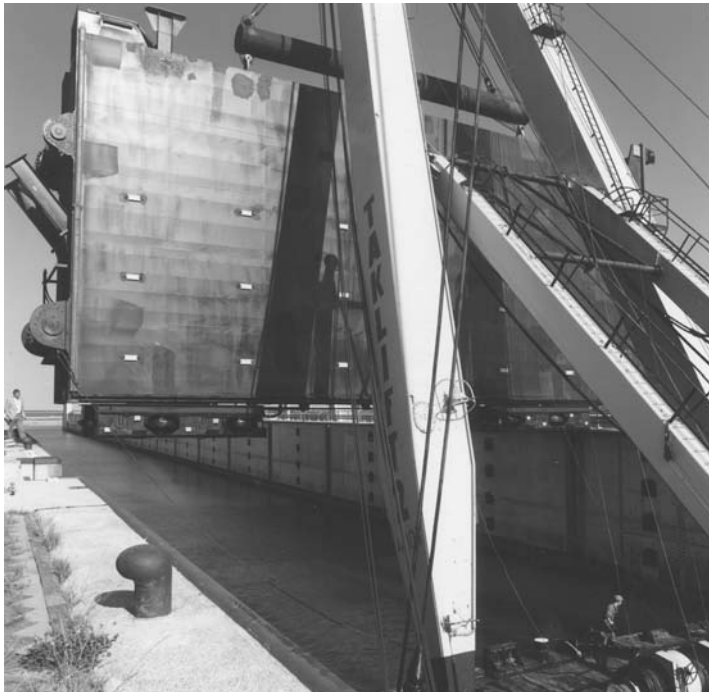
Photo 7.5 Rolling gate at Krammersluizen during installation (1985)
