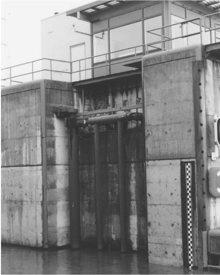
Photo 7.21 Frame shaped locking device for single pivot gate of the lock at Nieuwe Statenzijl
