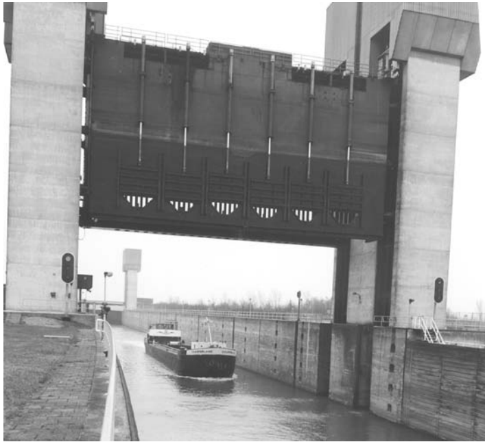
Photo 7.7 Lift gate at Prins Bernardsluis in Tiel
