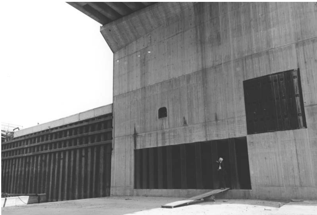
Photo 6.19 Outflow opening of the bypass culvert of the lower head of the locks at Maasbracht
