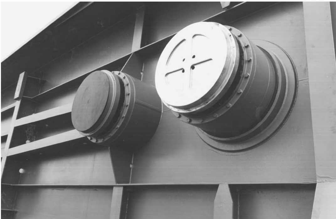
Photo 7.28 Fixed load bearing shoe and hydrostatic bearing of sliding gate of Nieuwe Oranjesluis in Amsterdam
