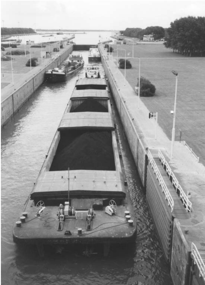
Photo 4.16 Pushed barge CEMT class Va
