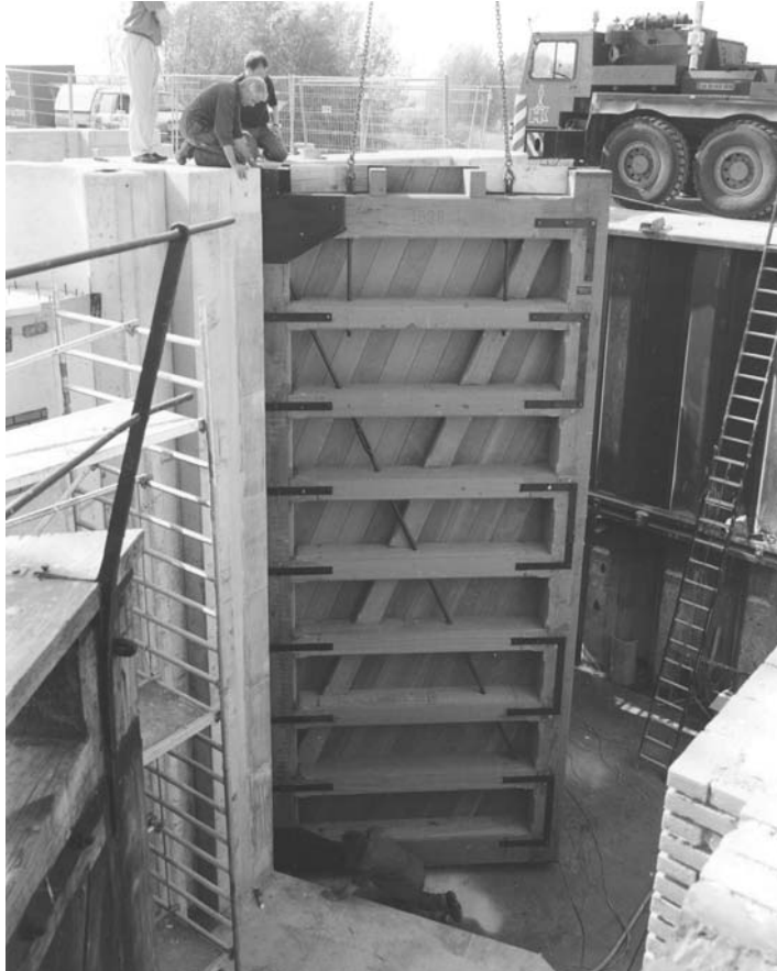
Photo 7.2 Wooden mitre gate of lock at Dalem during positioning (1998)
