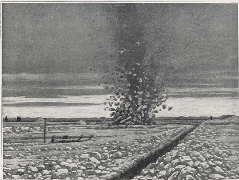
EXPLOSION DE TONITE
