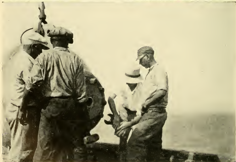
FIG. 67. ( upper ) The half-mile of solid rubber hose has now been unwound from its spindle and coiled loosely on deck. One weak spot has been cleverly spliced by a friend from the Wireless Station, and the four internal wires work perfectly, transmitting sound and light. A squall is approaching, making diving impossible, and the bathysphere is being lashed to keep it from rolling about. FIG. 68. ( lower ) Before a human goes down in the bathysphere it must be sent for a test dive, deeper than the intended descent. The 400-pound door is swung into place and fastened on.
