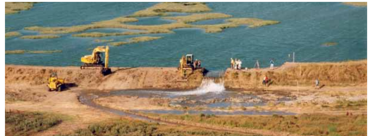
Figure 3. Tollesbury managed realignment site, Essex. The initial breach in 1995 showing the first seawater entering the site. Copyright Carol Reid 1995
