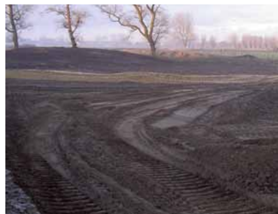
Figure 6. Final appearance after works (Dec 2004)
