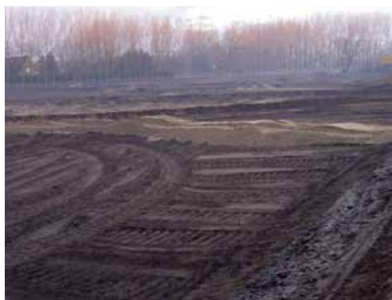
Figure 5. Embankment near the motorway (Dec 2004)
