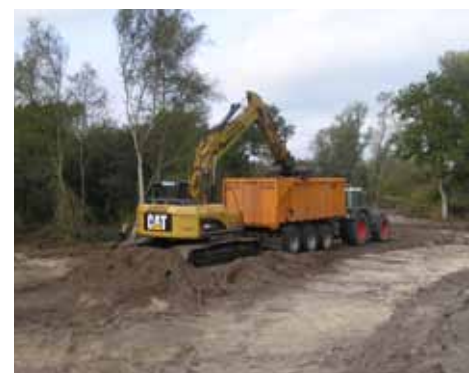
Figure 9. Cutting sods of grass in the western corner
