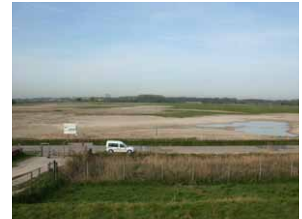
Figure 13. After the work (April 2010)
