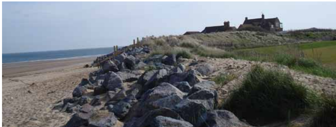
Figure 5. At Brancaster, North Norfolk, removal of rock armour on sand dune frontage led to restoration of dune and saltmarsh function as part of the Living with the Sea LIFE project in 2002. Copyright Angus Garbutt
