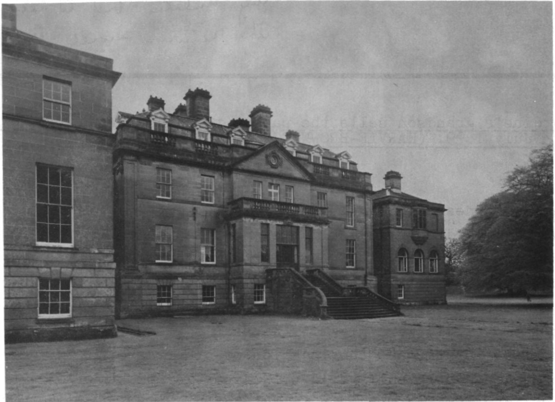
6. North view of Jardine Hall before it was demolished in 1964.
