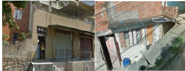
Figure 17 and 18: Typical Building Source: Google Earth, 2015
