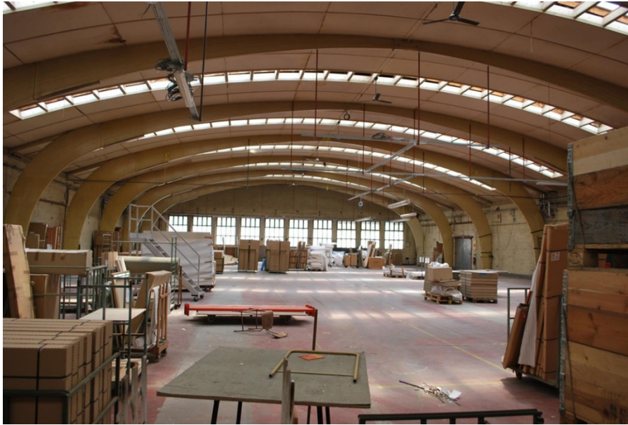
Figure 9, Reuse: the wooden construction in this warehouse proved to be an unique feature. The site is going to be reused as a covered farmers market in the nearby future.
