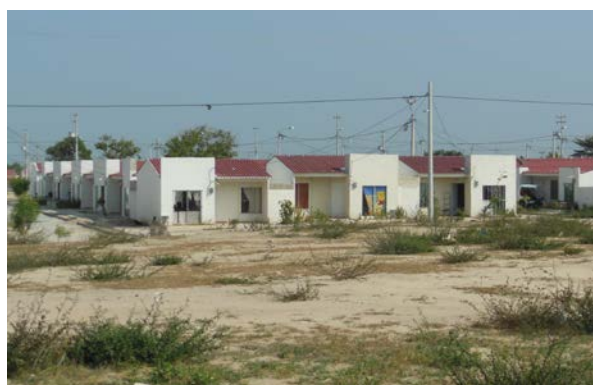
Figure 2. Nueva Esperanza housing project
