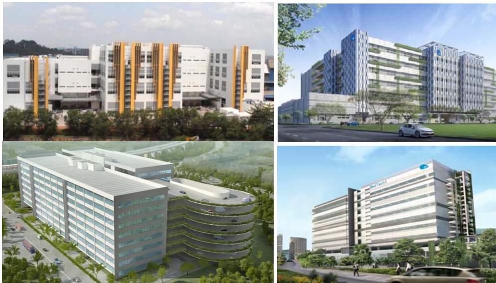
Figure 4: JTC Surface Engineering Hub, JTC Food Hub @ Senoko, JTC MedTech One @ MedTech Hub, JTC Furniture Hub @ Sungei Kadut (above left, clockwise) (Source: JTC Corporation)
