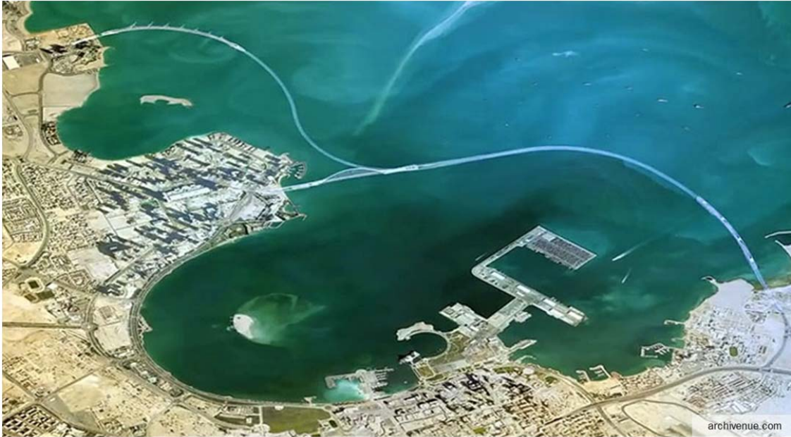
FIGURE 16 DOHA SHARQ CROSSING OVERVIEW SOURCE: ARCHIVENU.COM
