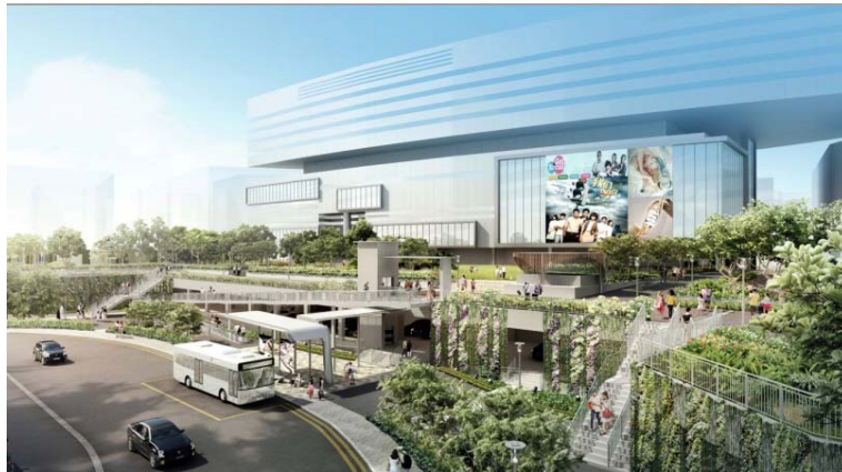
Figure 6: Multi-Utility Hub at one-north (Source: CPG Consultants)
