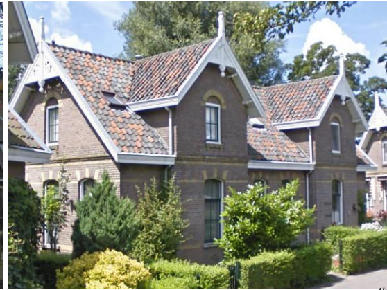
typical architecture of the first part built in de 19 th century
