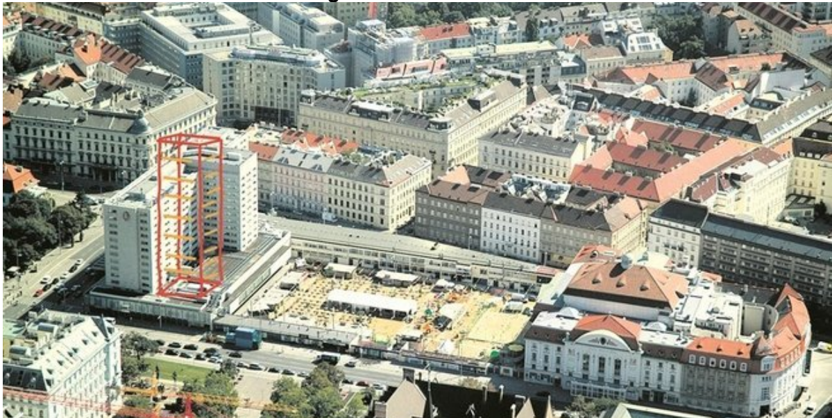
Fig. 7: “Eislaufverein” site with summer use and the proposed tower (red), Wiener Zeitung, 11.7.2013
