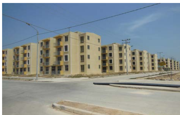
Figure 1. Villas de San Pablo housing project
