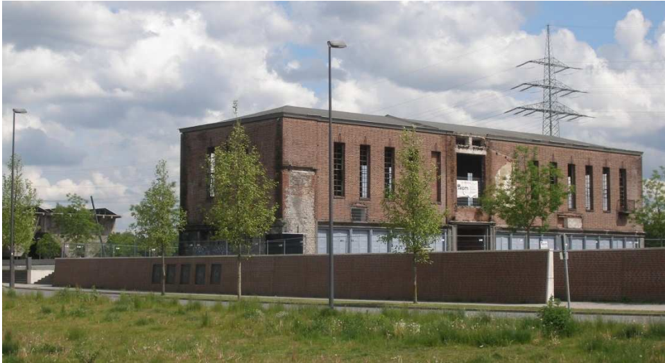
Figure 4: One of the abandon buildings on the site of Schalker Verein. View from the Kesselstr., June 2014 (source: author)
