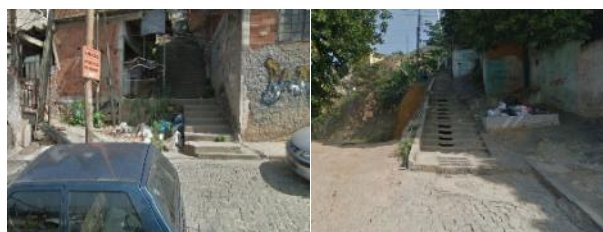
Figure 13 and 14: Slip risk areas. Source: Google Earth, 2015
