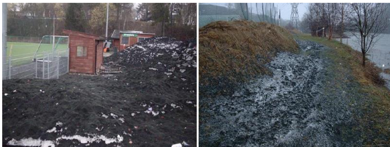
Figure 21 – Infill Accumulation from Snow Removal in Norway
