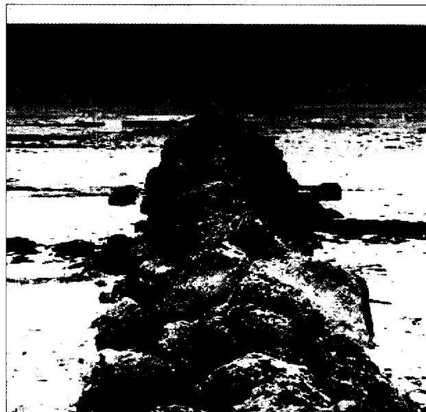
Plate 27: Groynes constructed of granite blocks on the shore of Anse Kerlan, Praslin, Seychelles
