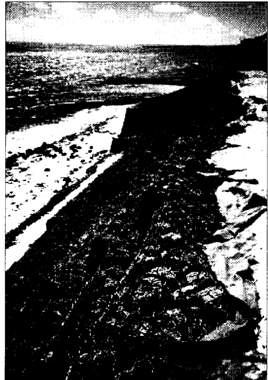
Plate 24: Rock-filled wire gabions form a defensive revetment on an eroding shore in Mauritius
