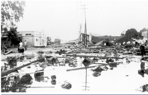
Destruction along the waterfront of Hilo, Hawaii, from the Pacific-wide tsunami generated off the coast of Unimak Island, Aleutian Island, USA on 1 April 1946.
