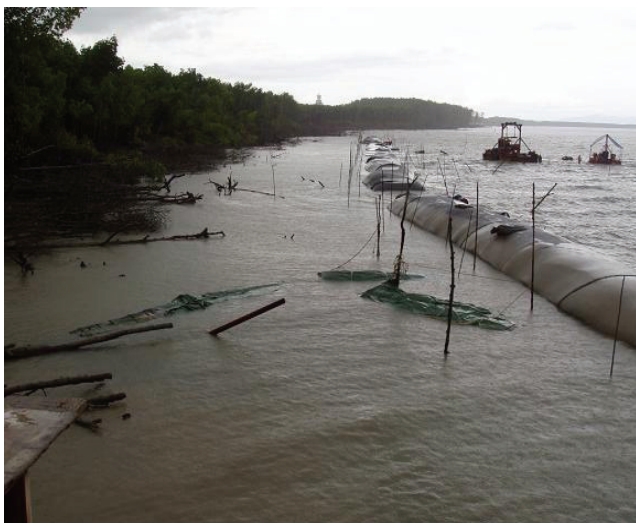
Sand-filled Geotextile tubes placed in front of eroding mangrove shoreline
