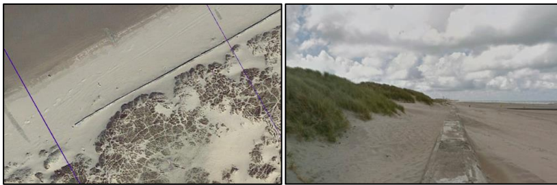
Figure 3-17. Concrete wall as a dune foot protection measure in section 72.
