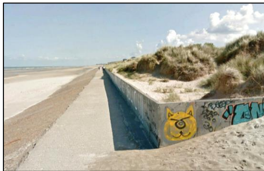
Figure 3-13. Concrete revetment and wall, built to reinforce the dune foot in section 8.
